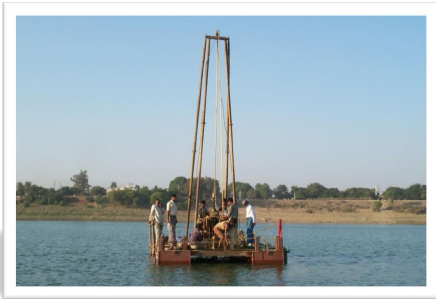
Drilling work in progress at Cable stayed Bridge at Naini, Allahabad
